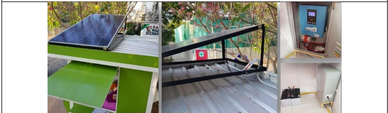
Solar PV Power for Electricity in a Waste Bank (ARU, Thailand)
