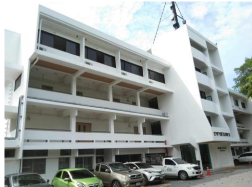
Building Renovation (ARU, Thailand)
