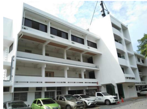
Building Renovation (ARU, Thailand)
