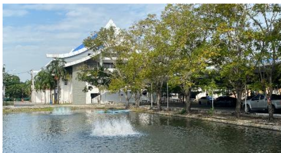
Aeration Lagoon (ARU, Thailand)
