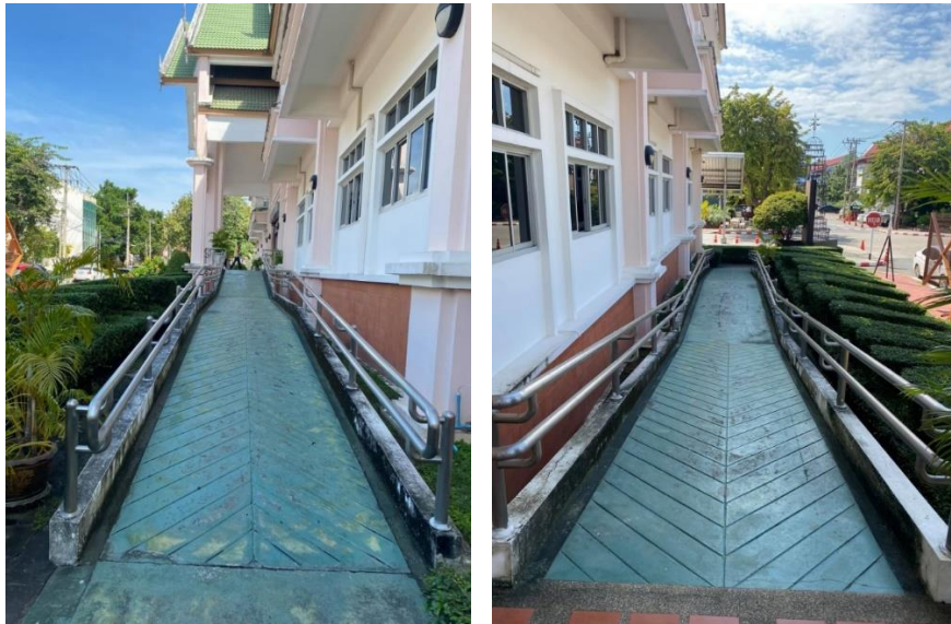
Wheelchair Ramp (ARU, Thailand)
