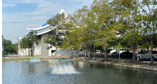
Aeration Lagoon (ARU, Thailand)
