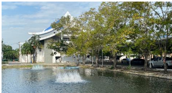
Aeration Lagoon (ARU, Thailand)
